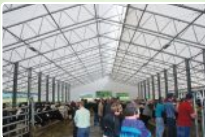
The latest expansion at Cedarbrink Farms consisted of a six row We Cover barn, built for light. The steel and tarp for the 150 x 128 foot barn went up in eight days, and has Cedarbrink's own uniquely designed comfort stalls in use.
