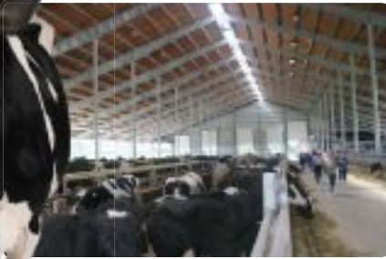
Lots of fresh air and light in the magnificent steel framed drive through barn at Klood Farms.
